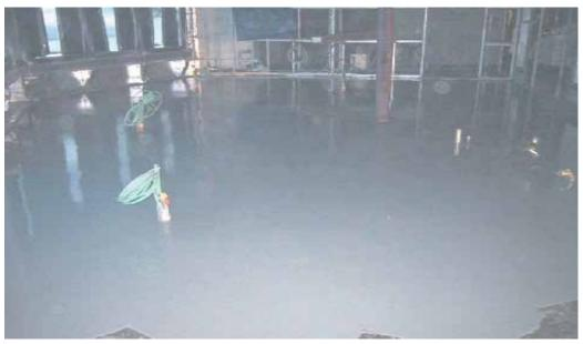
4. After app. 3-4 hours at 20°C. the floor is ready for walking and after 18-24 hours at 20°C and in a thickness of app. 8 mm. the floor is ready to be covered with carpet, PVC or tilling
