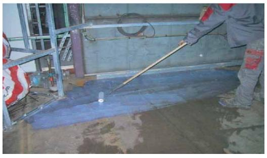
Spread out the primer 54 smooth in a thin a layer at the floor Approx. 0,1 kg. / m<sup>2</sup>
